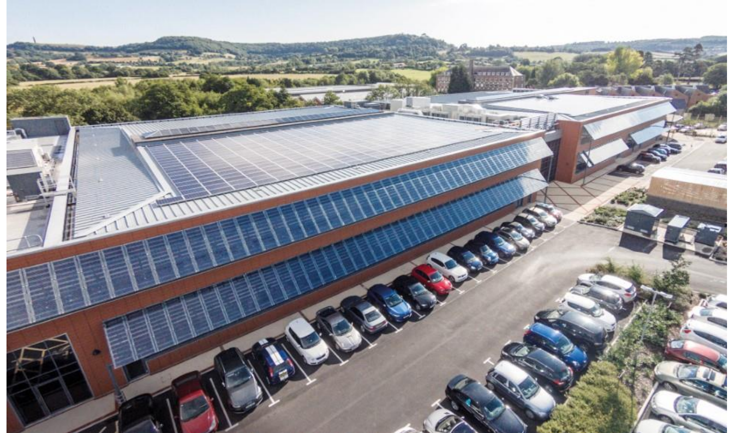
Solar panels on the Renishaw Innovation Centre at our UK HQ site
